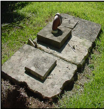
Existing concrete septic tank prior to upgrade
