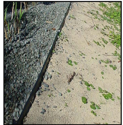
Stormwater diversion along reedbed edge
