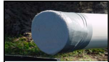
Geotextile covered ends
