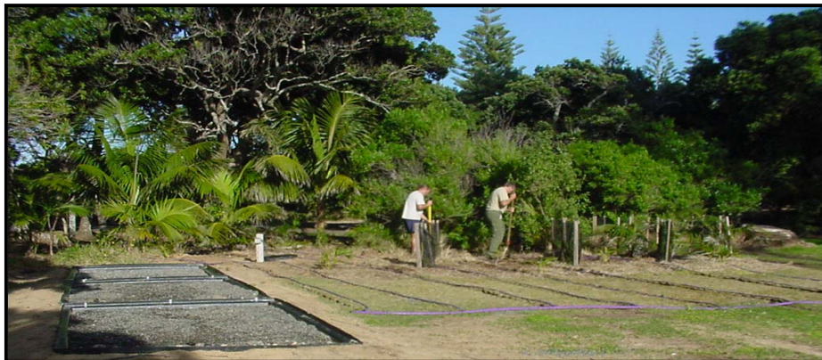
Laying irrigation grid
