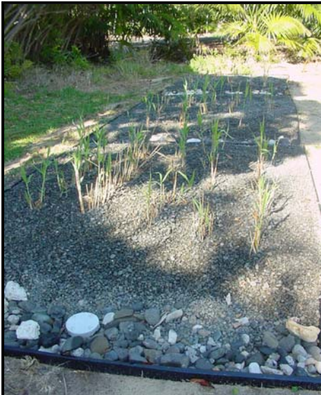
Reedbed fill of medium rocks and gravel
