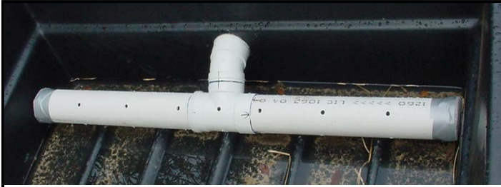
10mm perforations on outlet T
